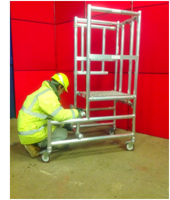
4) CLIP UPPER BRACE OF LADDER ABOVE RINGS ON VERTICALS WITH ASSEMBLED HOOKS AT TOP
