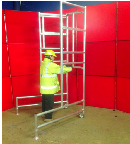
1) OPEN FRAME AND LOCK MECHANISM
