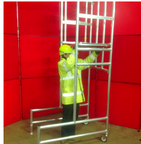
2) FIT PLATFORM AT CORRECT HEIGHT
