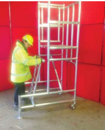
4) CLIP UPPER BRACE OF LADDER ABOVE RINGS ON VERTICALS WITH ASSEMBLED HOOKS ON TOP
